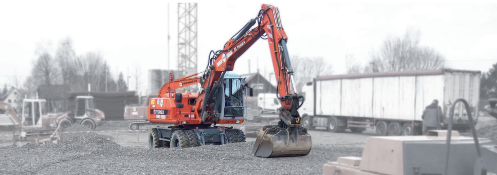
Extensive installation of GEOMATERIALS Foam Glass for a production hall
