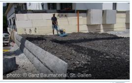
**GEOMATERIALS Foam Glass** interlocks itself, does not roll and therefore can be installed at inclined surfaces up to 15°. Due to the high friction angle, a modelling of slopes up to 45° is possible.
