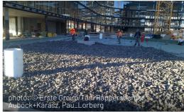
Despite the lightness, it remains stable because the foamed grains are closed-cell and thus do not absorb any water. The material interlocks itself, is resistant to pressure and therefore reduces the slope pressure. At the same time, sloping water can drain off easily.
