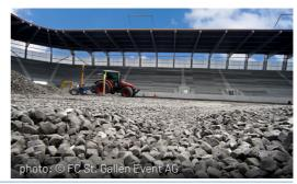
**GEOMATERIALS Foam Glass** not only reduces the surcharge with only 150 kg/m<sup>3</sup>, but it also has higher compressive strength with simpler and less expensive installation technique.
